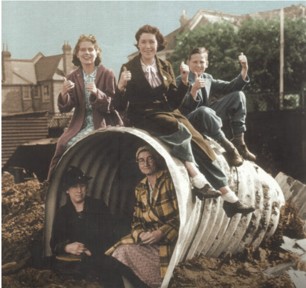
ABOVE: dirt cheap countermeasures worked against blast. Earth cover was blown off this Anderson shelter in London during the 1940 Blitz. This damage to the shelter absorbed blast energy, permitting survival inside, just as car bumpers and "crumple zones" absorb impact energy and thus afford protection. Tables indoors offered similar protection against house collapse and flying debris.
